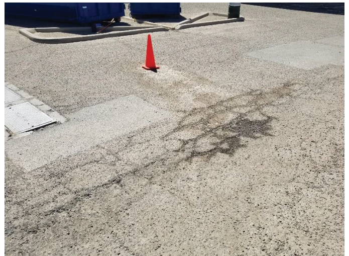
Photo No. 6: Alligator cracking typical.
